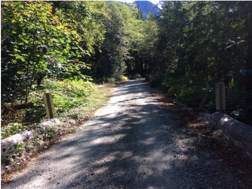
Left approach viewed from bridge
