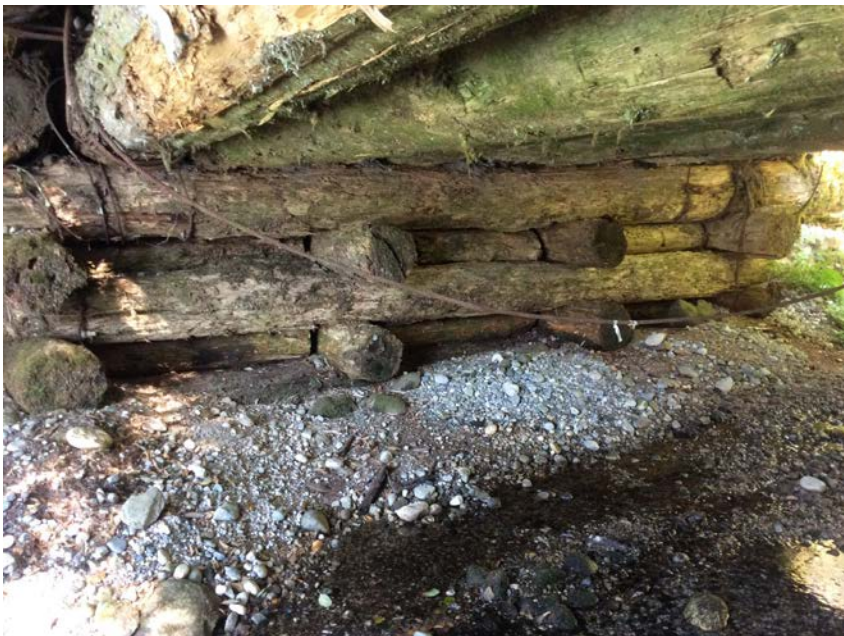
Right Bank Abutment when facing downstream
