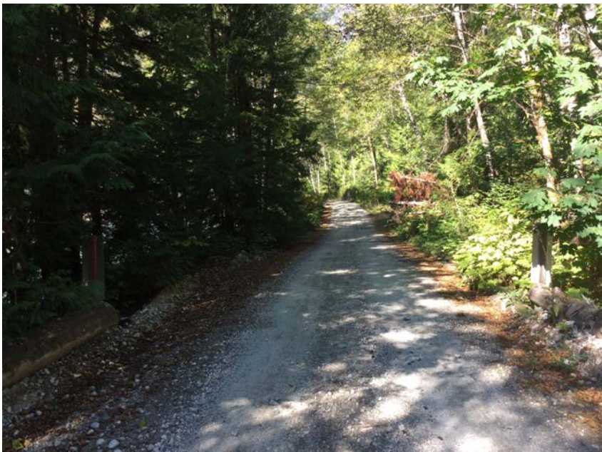
Right approach viewed from bridge
