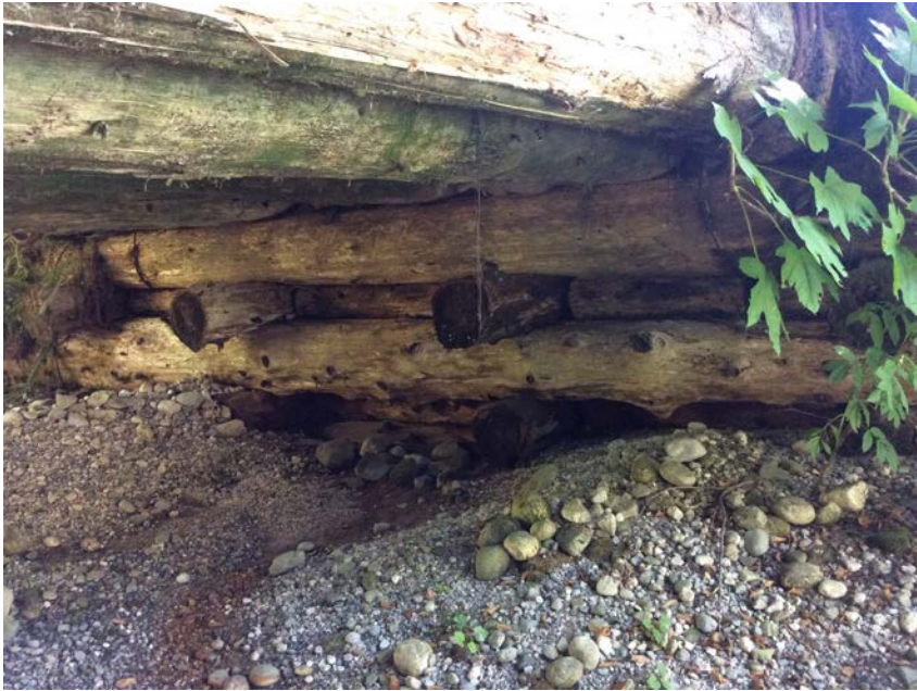
Left Bank Abutment when facing downstream
